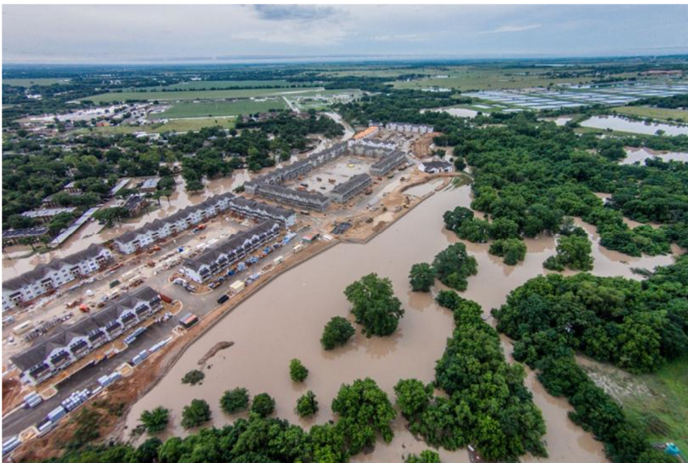
Figure 1-10: Memorial Day Flood Source: Stephen Ramirez
